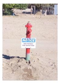
A new hydrant has been installed and connected to the old piping from the Tanganda well allowing for the use of the Tanganda well and storage tank to be used for fire and construction water. This well was removed from service as a drinking water well due to high arsenic and nitrate levels. The reconfigured facilities are completely separate from the drinking water system and the sale of construction water is anticipated to add an additional revenue stream to District operations.
