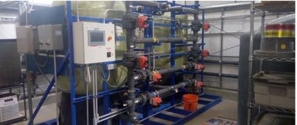
with the distribution SCADA system to automate the filtration system operation.
